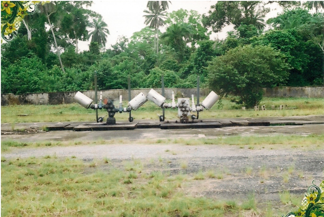
Oil well head in Etelebou flow station
