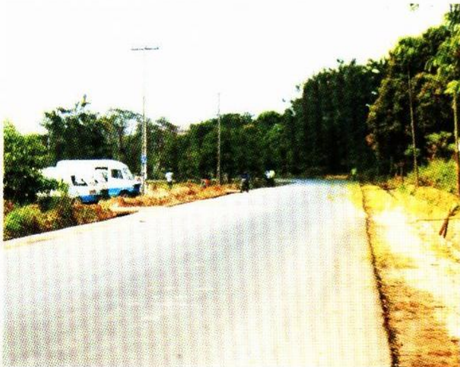
Road work in progress.
