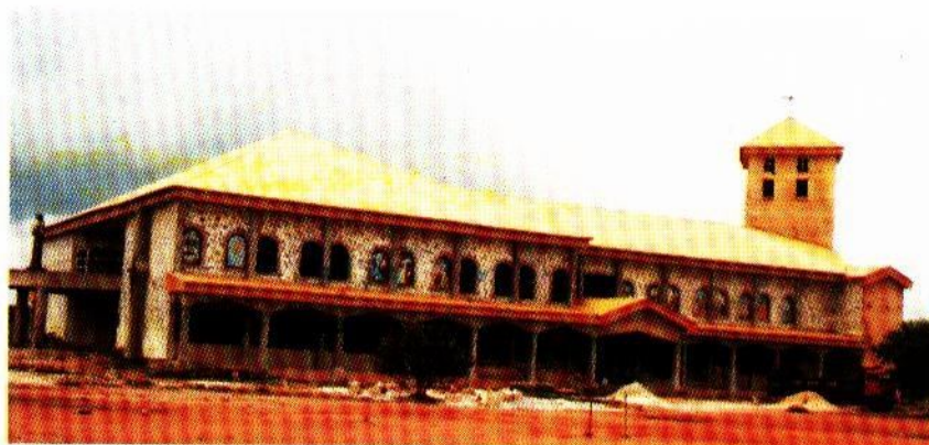
The St. Thomas Aquinas Catholic Chaplaincy (STACC) FUTO nearing completion.
